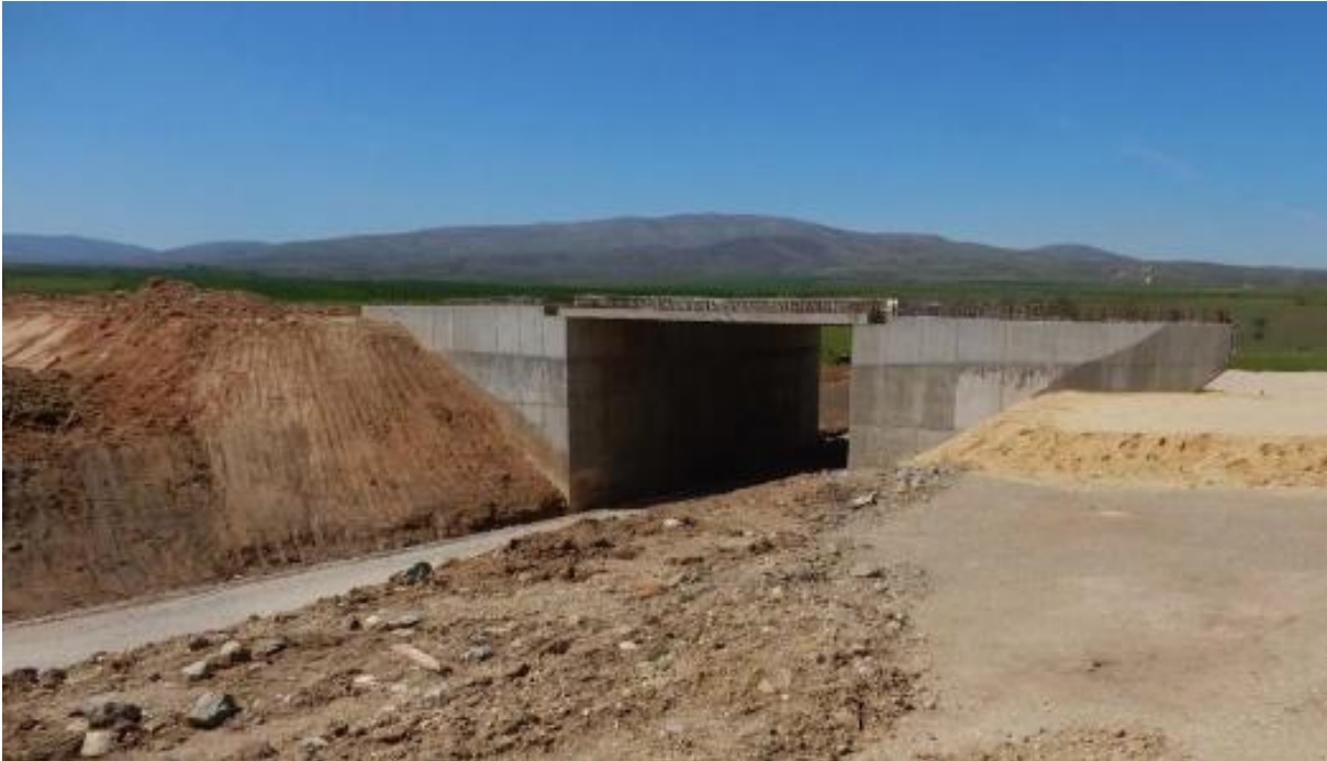
Source EIB: Construction of express road A1, Section Gradsko - Drenovo
